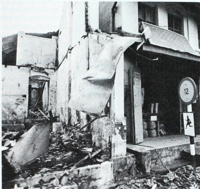
The burnings were very selective and accurate, clearly the product of highly organized planning. Some blocks of shops were completely untouched. In other blocks, many of the structures were gutted, often with undamaged Sinhalese-owned shops on either side of those burned.
